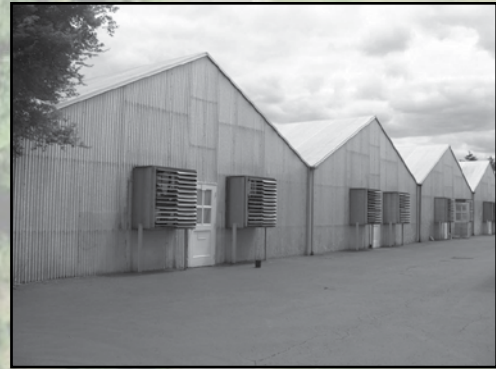
2009 photograph of the greenhouses at the Green Thumb Facility.
